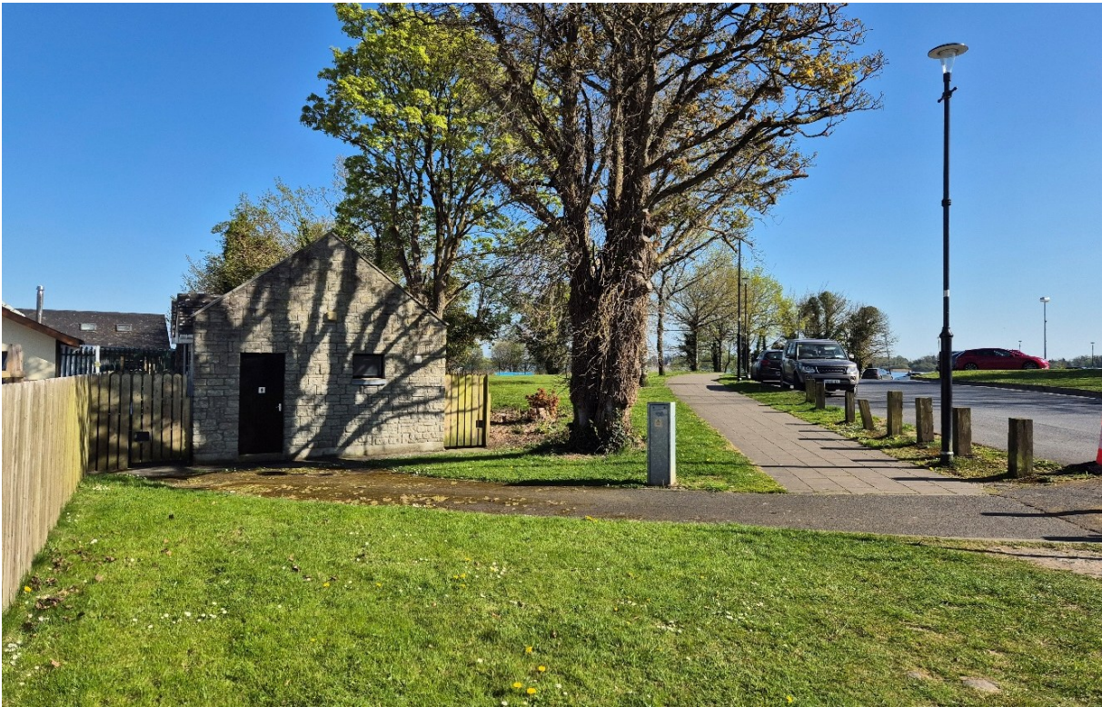
Plate 5 View of the existing toilet block on site for demolition looking Southeast
