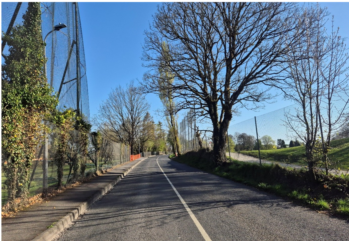
Plate 15 View of the L2020 Local Road and golf course boundary netting looking South
