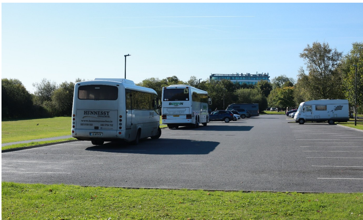
Plate 12 View of the Northern Carpark (Carpark C) on site looking South
