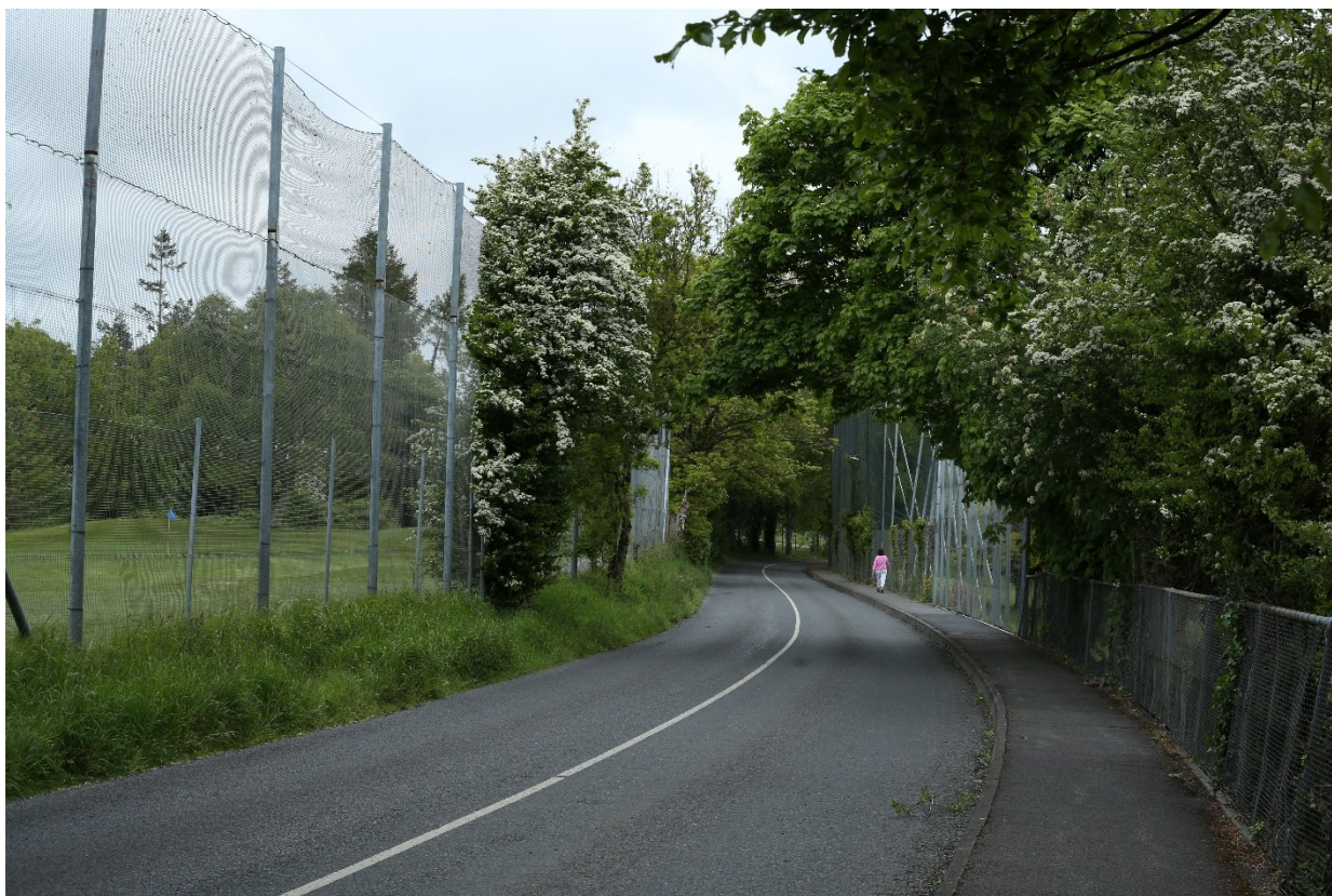
Plate 14 View of the L2020 Local Road and golf course boundary netting looking North
